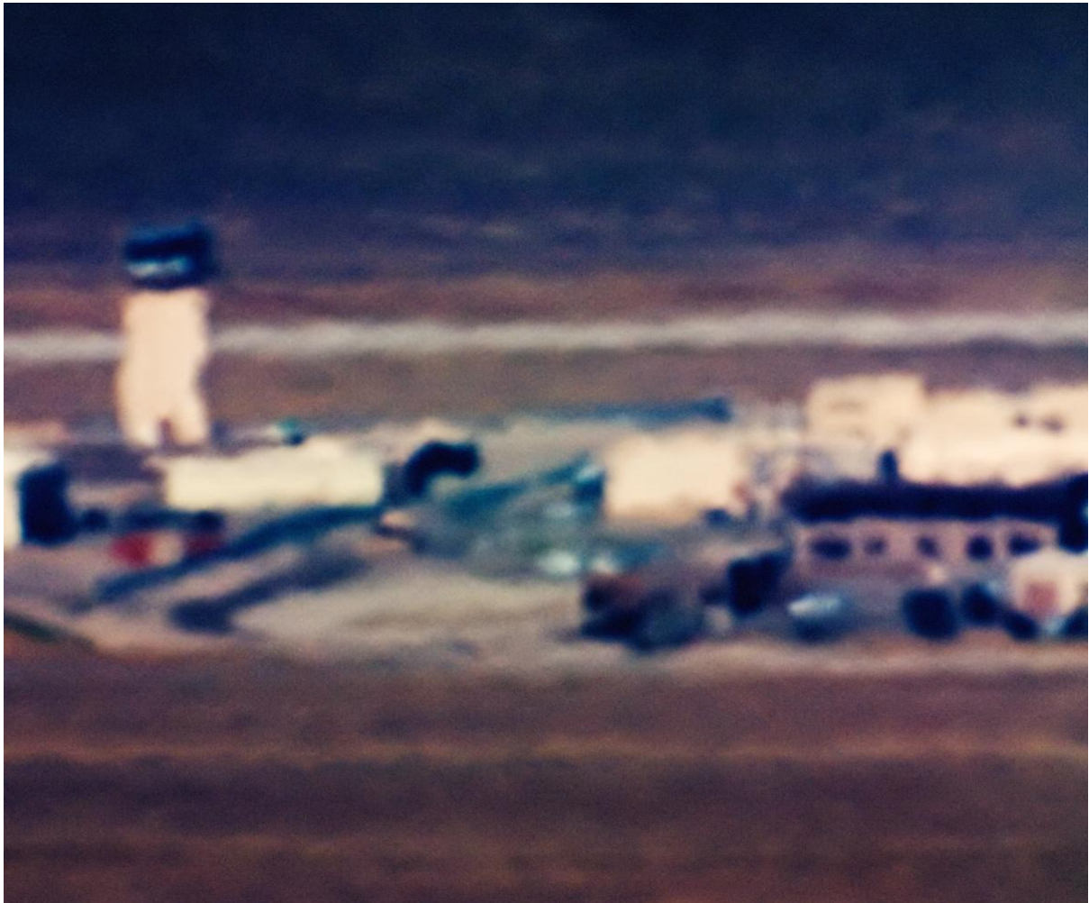
Control Tower (Area 52); Tonopah Test Range, NV; Distance ~ 20 miles; 11:55 a.m., 2006
